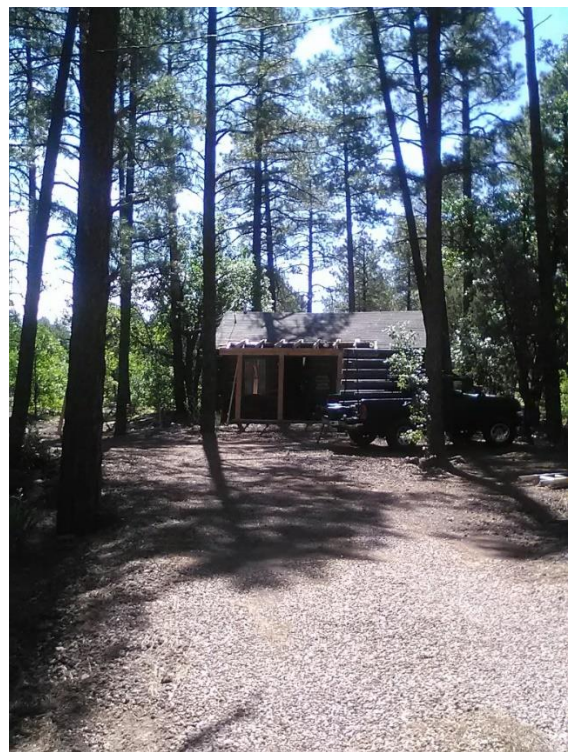
Porch being built
